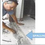
SPALLING = CONCRETE CANCER Spalling breaks up the concrete under track and interior and exterior concrete areas as well. DO NOT IGNORE SPALLING- VERY SERIOUS!
