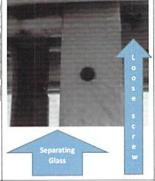
Corroding & rusting screws break or back out causing GLASS SEPARATION.
